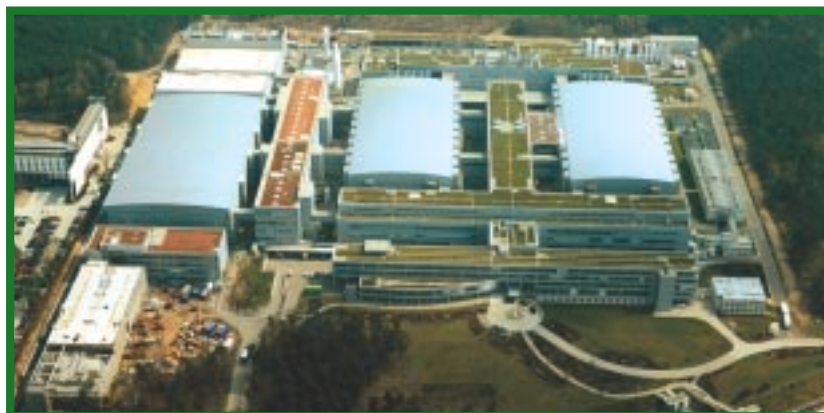
Figure 1. The picture shows the new 300mm fab complex (left hand side, front to back: Office buildings, Fab, Central Utility Building) and the 200mm Fab modules (middle and right hand side). The Support Building between the old and new Fab module was extended for process and testing activities.
